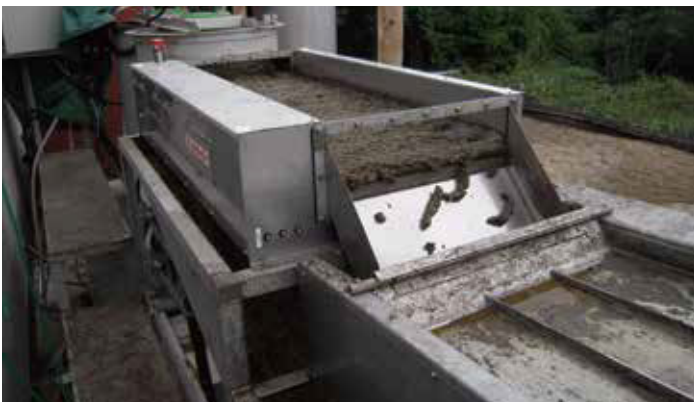
Pig dung wastewater treatment
