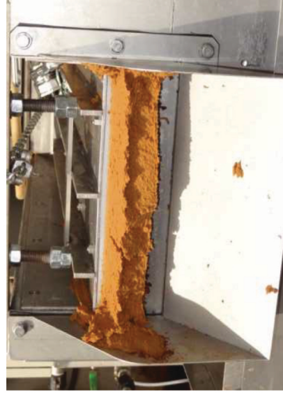
Purified water tank grime
